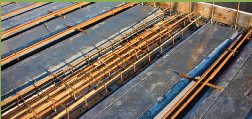
Typical Floor Installation with insitu beam
