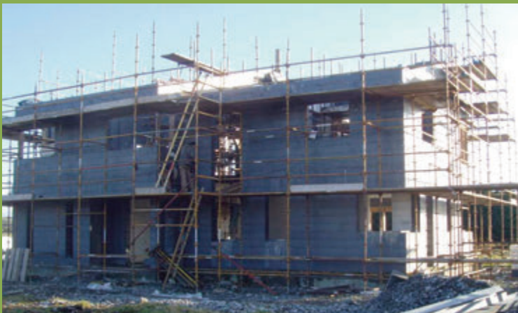
Two Storey Construction
