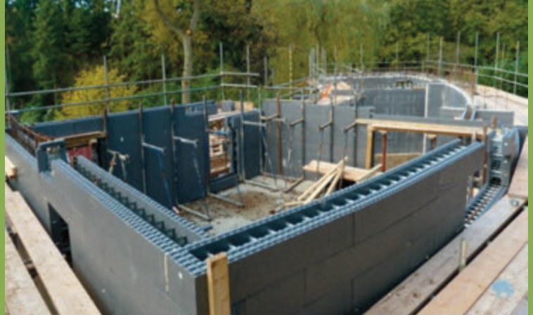
ICF Curved Wall Construction
