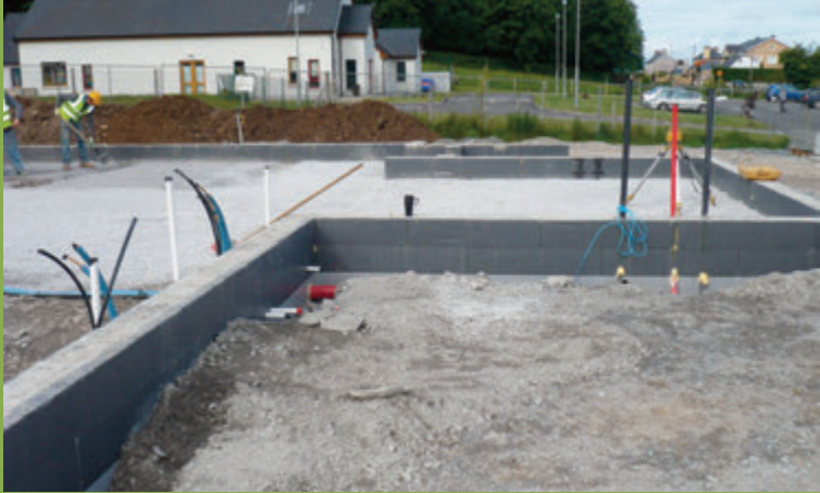
Thermohouse ICF Rising Walls / Dead Work
